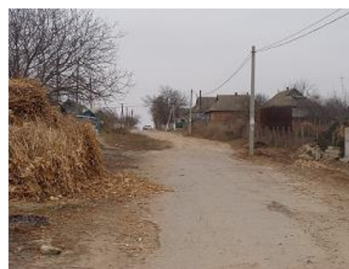
Fig.3: Road from Carahasani village before rehabilitation.
